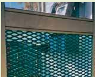
▼ Plascoat® PPA 571 coating still as new after 6 years.
