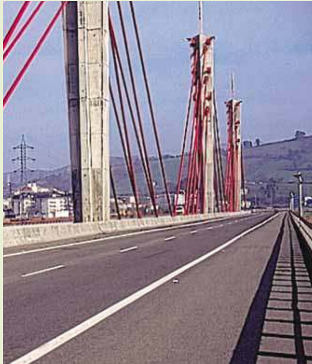
► Suspension cable covers after 10 years in northern Spain.
